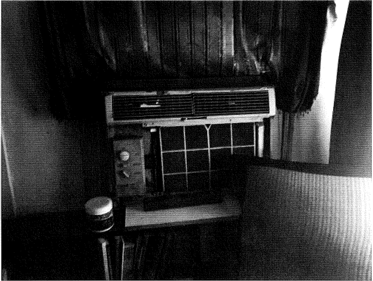
Entry Room AC
