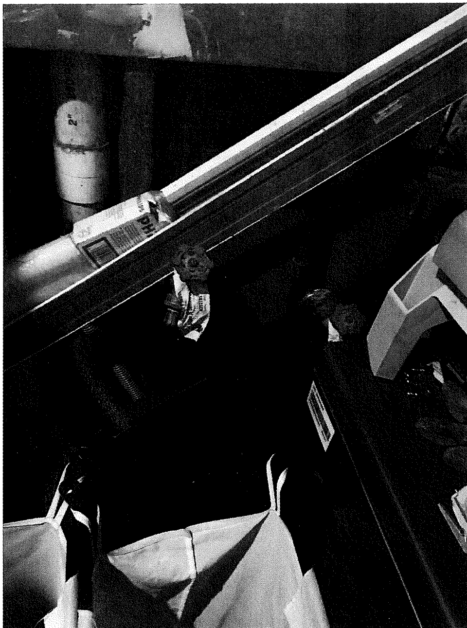
Drywall missing at Laundry Room
