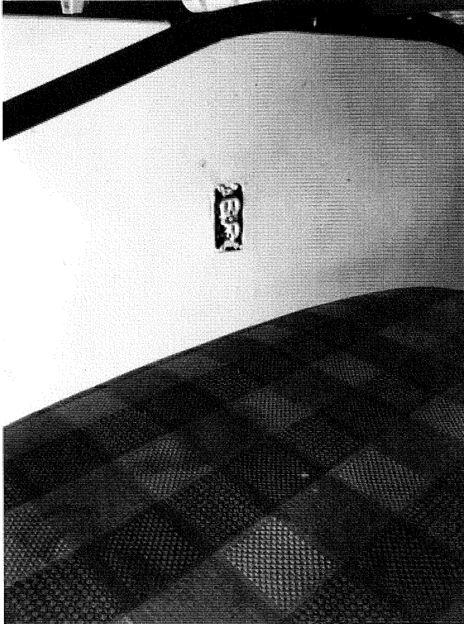
Damaged Receptacle
