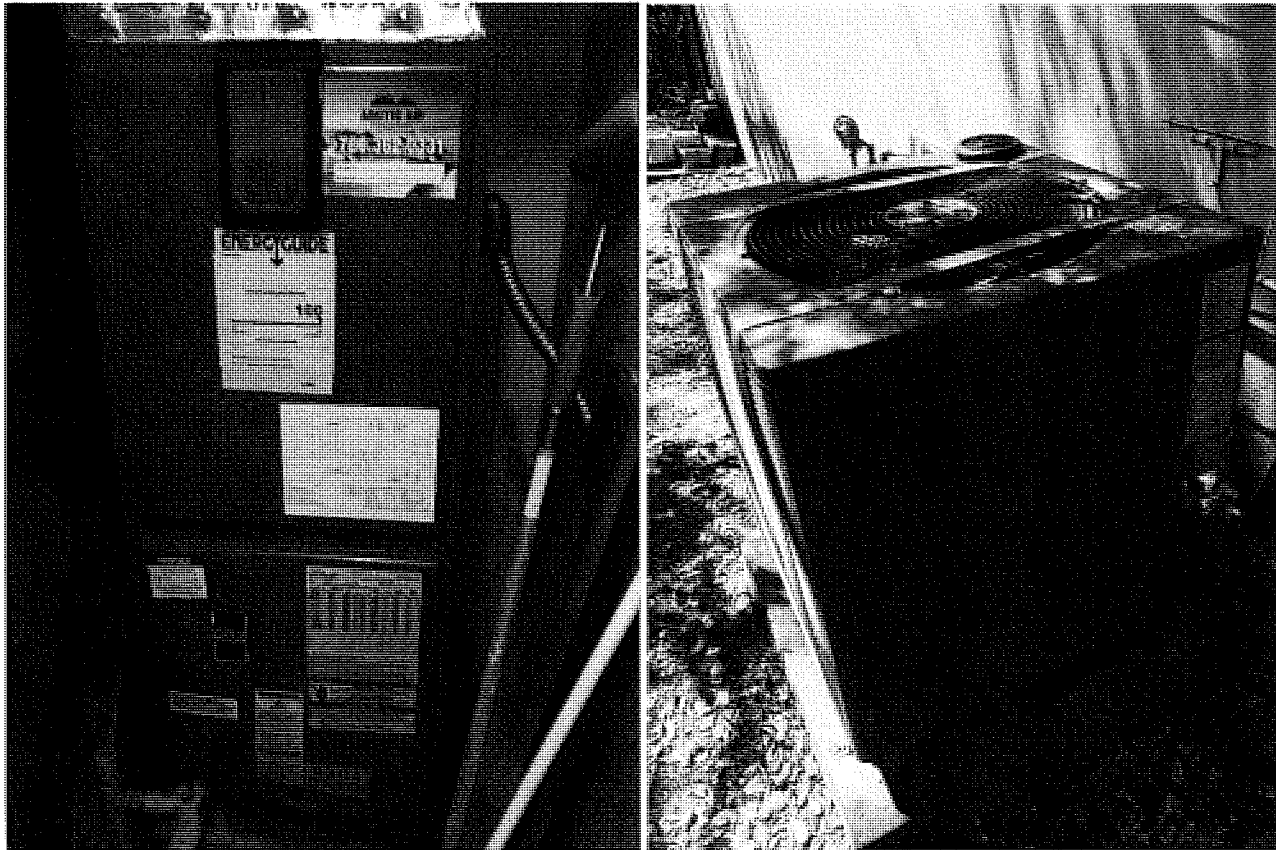
Left: Fan Coil Unit; Right: Condensing Unit
