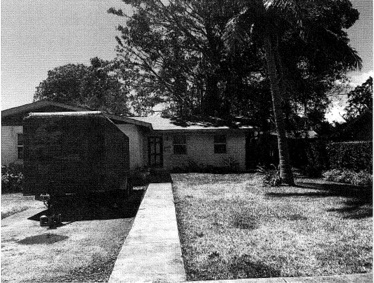
Front Elevation showing only a layer of underlayment roofing material installed
