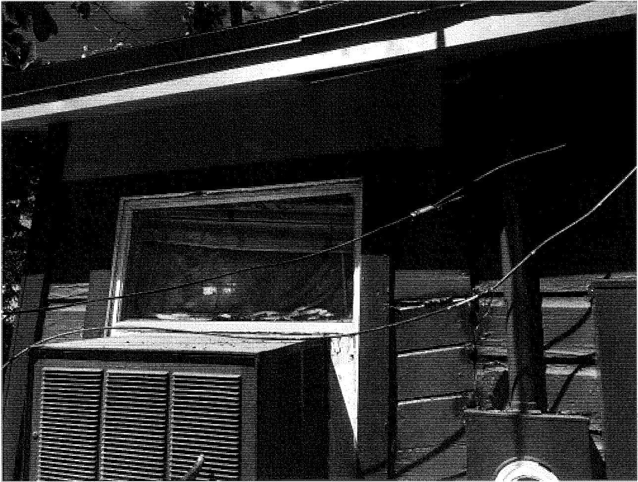
Exterior View of Entry Room AC. Note the poor construction of the walls.
