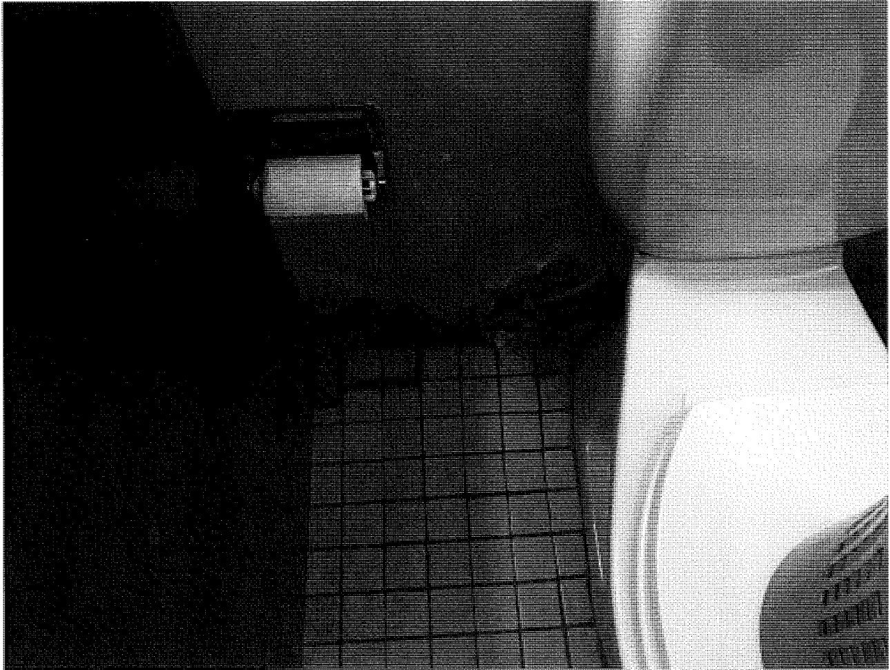
Damaged Wall at Master Bathroom
